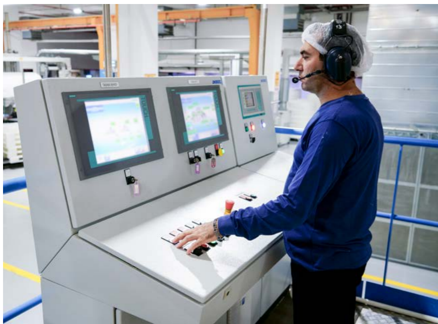
Monitoring system for process supervision
