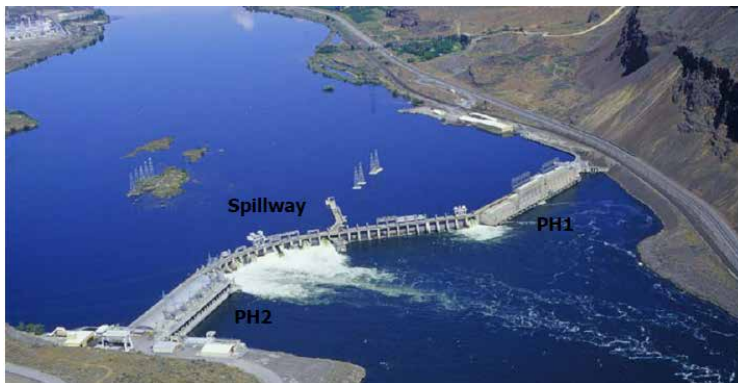
Rock Island power plant 18
